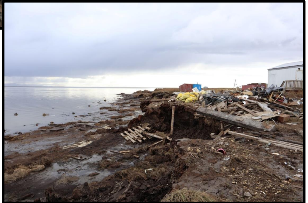
Storm debris and coastal erosion, Newtok, AK
