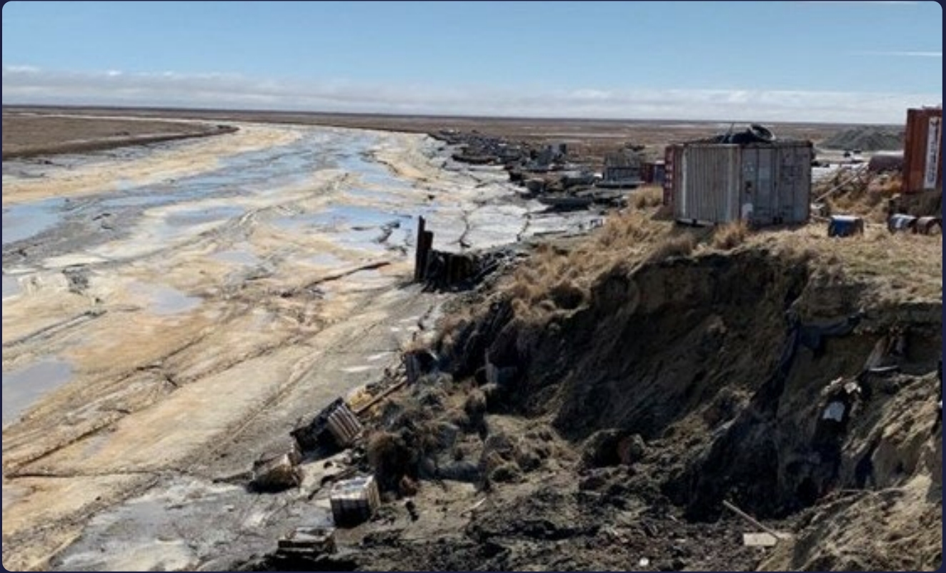
Image 1: Eroding Barge Landing, Chevak, May 24, 2023
