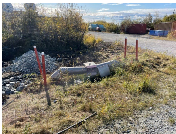
Image 17: One of Few Examples in Koyuk of Above-Ground Water Pipes, September 12, 2023
