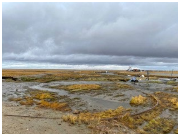
Image 21: Bent Fuel Line Due to Ice Scammon Bay, September 27, 2023
