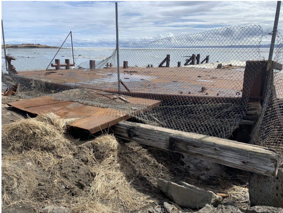
Image 19: St. Michael Barge Landing, May 2023
